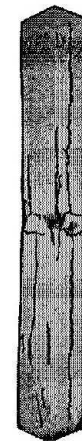
Fig. 5 : Mode of failure and crack pattern of columns with precast ferrocement jackets divided into two halves
