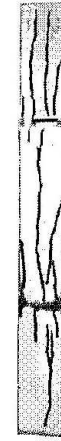
Fig. 6 : Mode of failure and crack pattern of columns with precast ferrocement jackets divided into three segments
